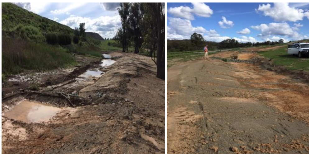
Plate 6 Maintenance of Bund Wall / Overburden Emplacement Area Drainage System
