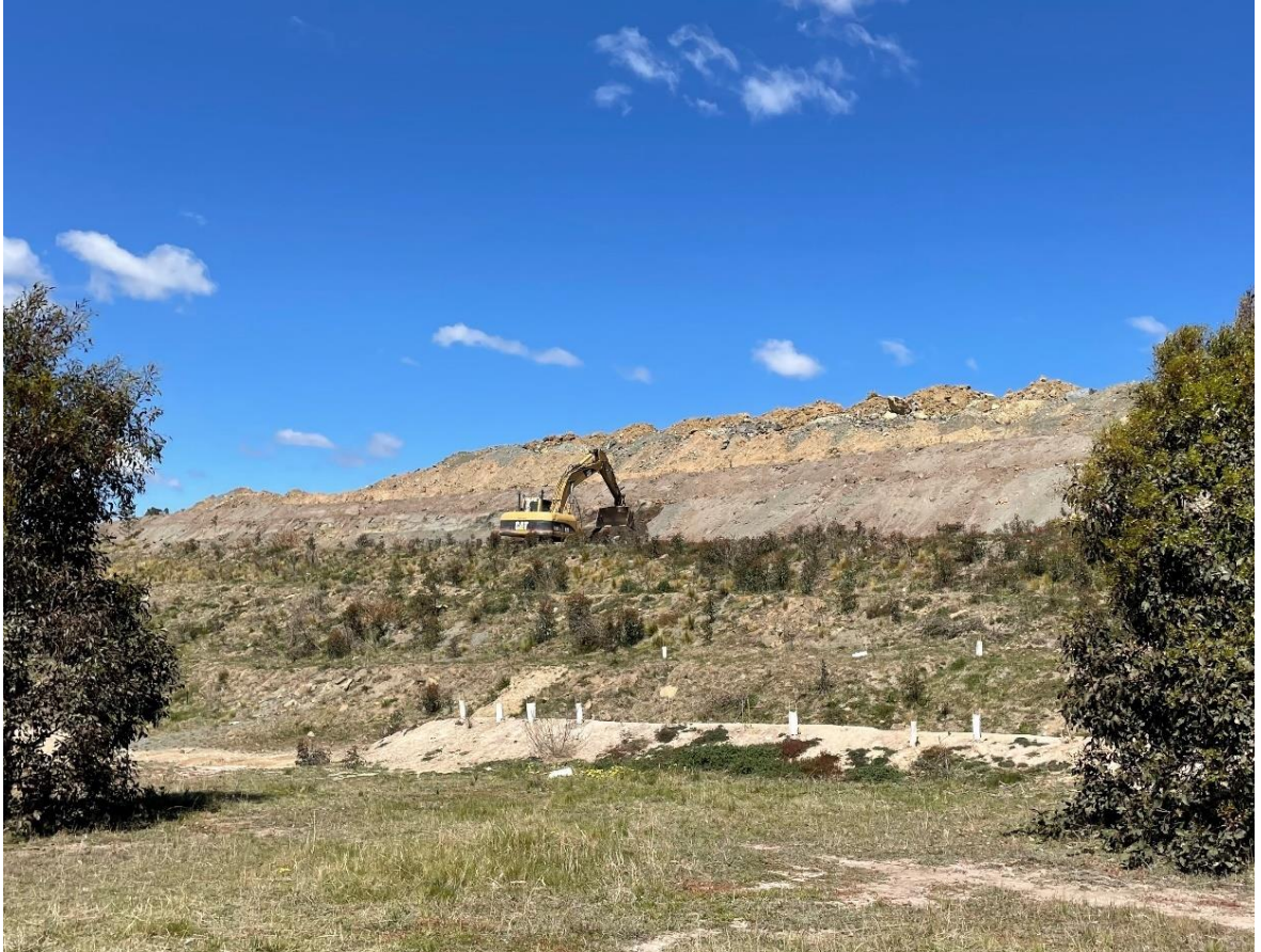
Plate 10 Rehabilitation Works Western Overburden Emplacement Area
