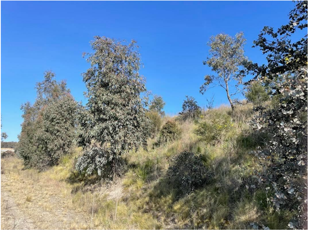
Plate 8 Rehabilitation of Bund Wall
